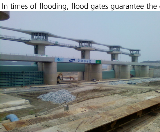
Fig 1: Floodgates under construction
